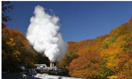
Gambar 5. Kakkonda Geothermal Power Plant, Iwate, Japan [14].
